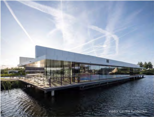
Visitor Centre Kinderdijk
